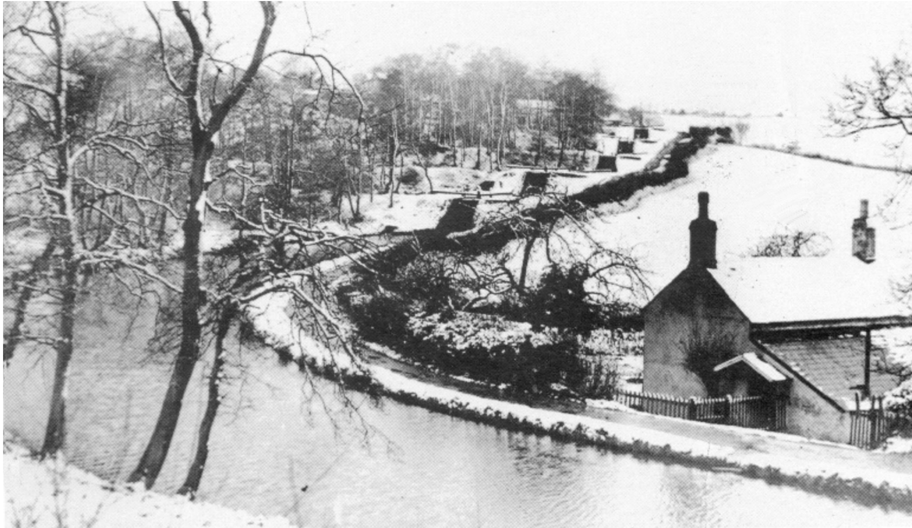
A snowy view of locks 8 to 12 in 1935 before the motorway was built.
