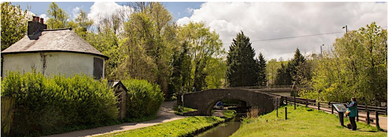
Junction House at Pontymoile
