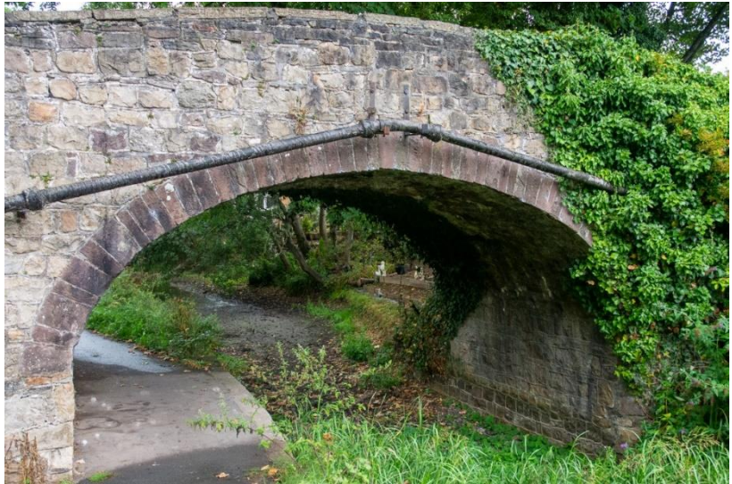
The canal at Rogerstone lacking water, summer 2022
