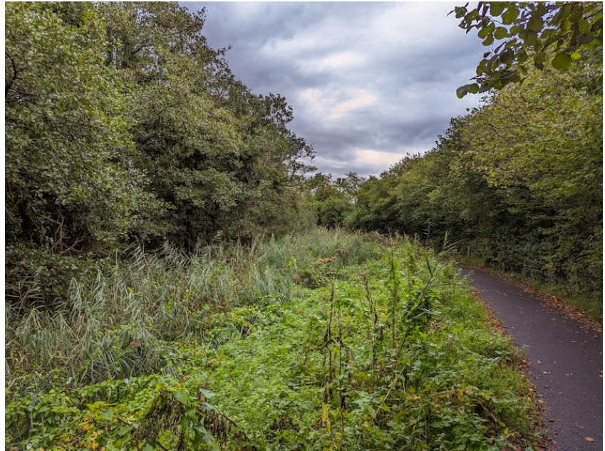
The canal full of weeds, and overhanging trees at Pentre Lane, north Newport
