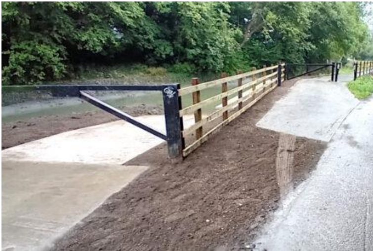
The finished slipway at Pontywaun
